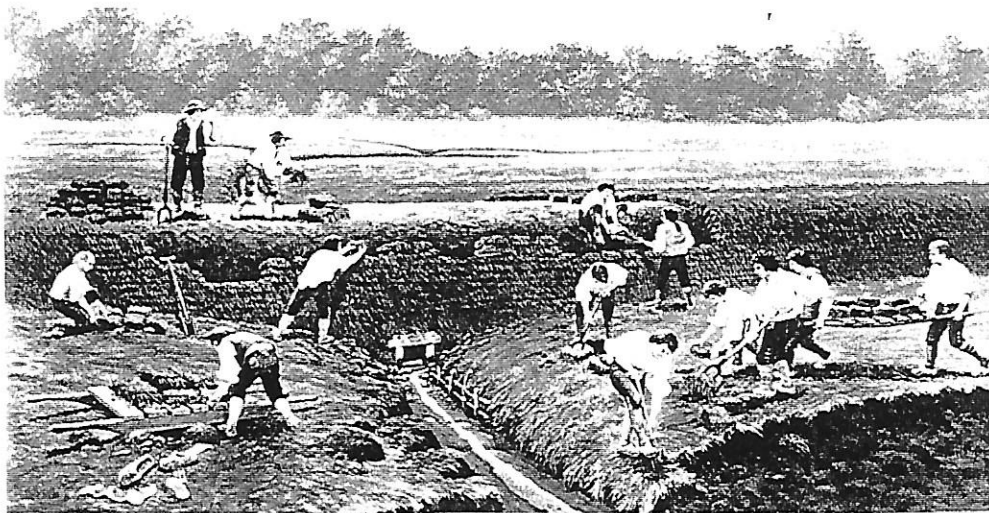
Figure 4. Acadians repairing a dyke (from a painting by Azor Vienneau) Nova Scotia Museum
